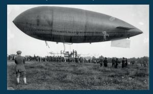
The airship balloons can be filled with hydrogen or helium, which are gases that are lighter than the air around them. As the balloon is lighter than the air around it, it floats.
